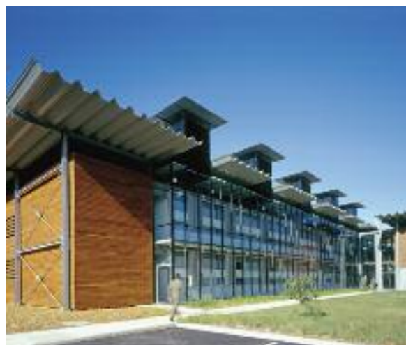
RAAF RICHMOND 36/37 SQUADRON HEADQUARTERS AUSTRALIA'S FIRST 5 STAR GREEN STAR BUILDINGS AND INTERIOR 2005
