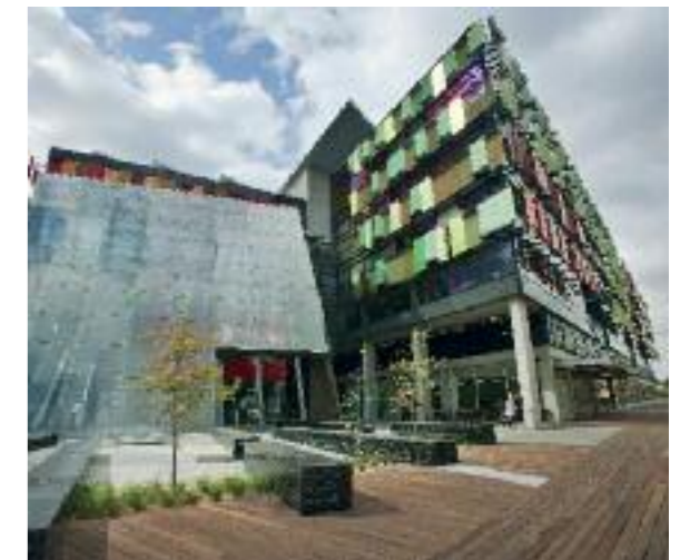
BENDIGO BANK HEADQUARTERS 5 STAR GREEN STAR REGIONAL BUILDING 2009
