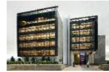
Sovereign Head Office New Zealand Completed 2007 Value $60M Client Northcote Road 1 Holdings Limited and Sovereign Services Full Architectural Service
